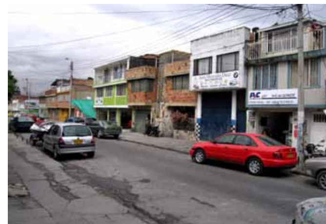
Self built, high density, owner-built housing in Bogota Colombia
