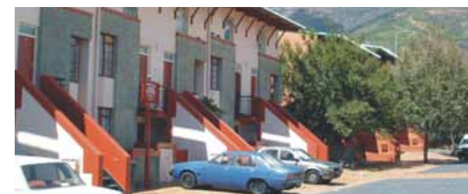
Springfield Terrance in Woodstock is an excellent example of how social housing can be integrated into an existing network of streets. Certain buildings have since been sectionalised and are now owned and managed privately
